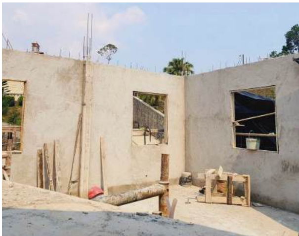
The new church offices are almost finished. They hope to be using them by August!
