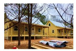
By God's grace, our goal of having both cabins "dried in" (framed, sided, doors & windows installed, and roofed) before the end of the year was met by mid-December. The upcoming phases include exterior painting and staining, as well as the plumbing, electrical, HVAC, and insulation installations.
