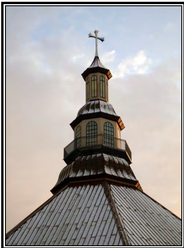
Our Savior Church Steeple
